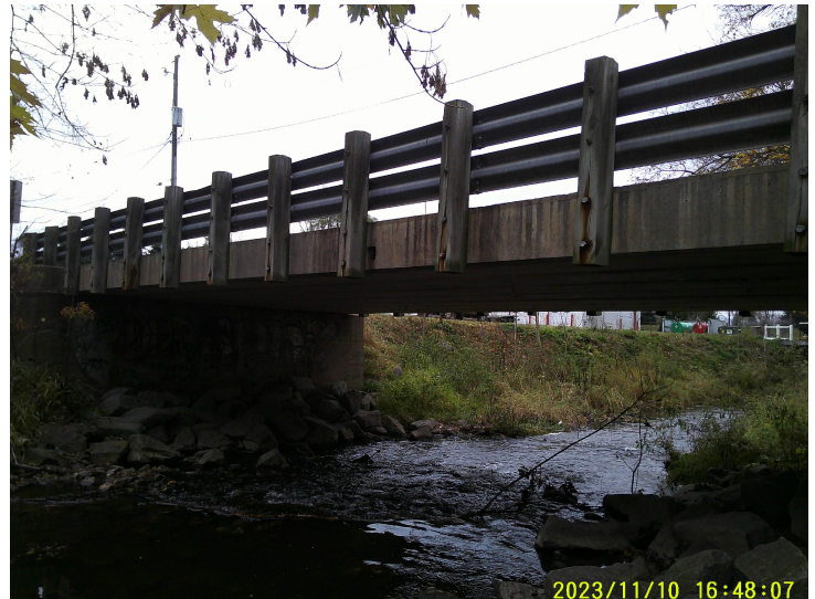
Document Name: DSCF0035.JPG Category: Railing Span Number: Comments: West railing, split posts
