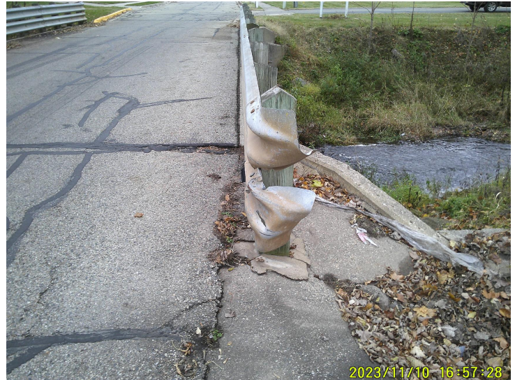
Document Name: DSCF0045.JPG Category: Railing Span Number: Comments: Bent ending on east rail, south end.
