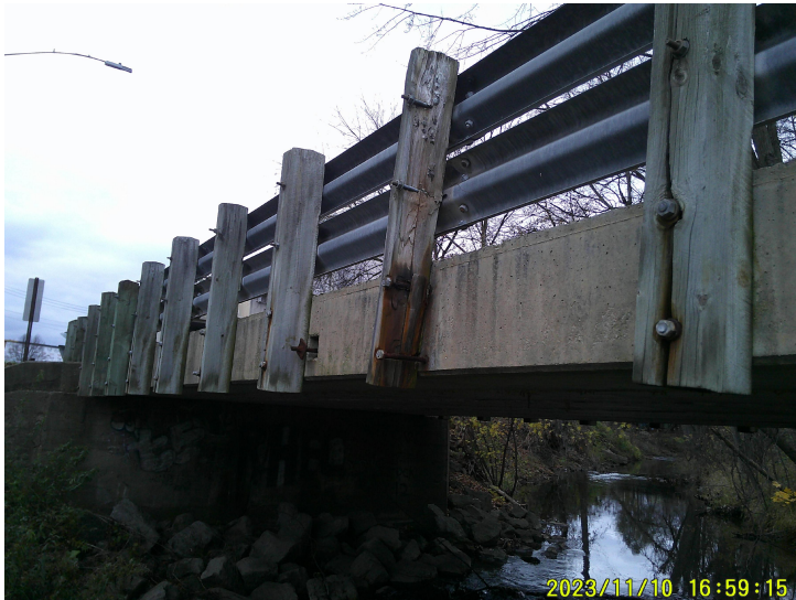
Document Name: DSCF0046.JPG Category: Railing Span Number: Comments: Split post on east railing, north end. Loose Post tension rod.
