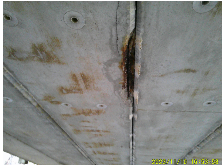
Document Name: DSCF0040.JPG Category: Superstructure Span Number: Comments: Beam 3W at 1/3 span, spalled with exposed strand
