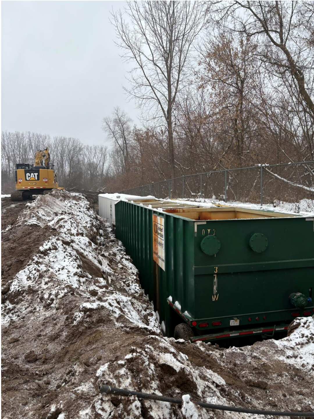
Frac Tanks Placed in Excavation
