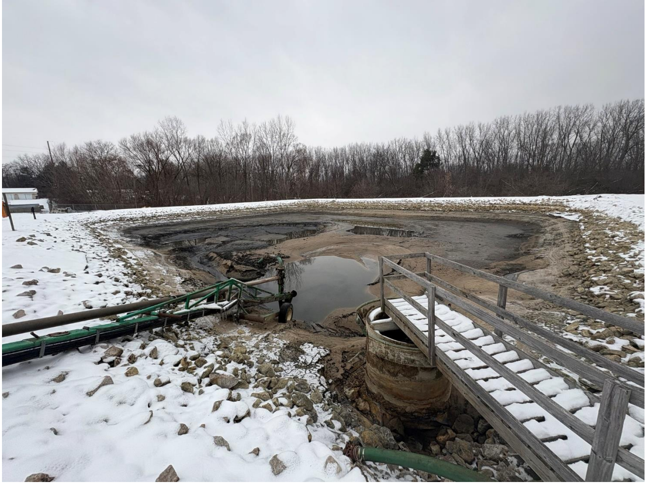
Biosolids and Water Removed from Polishing Pond
