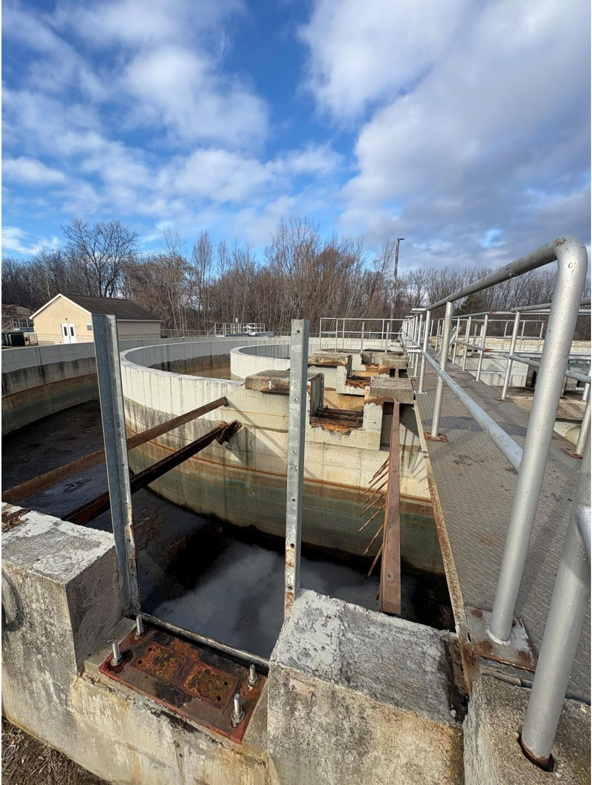
Oxidation Ditch Demolition Progress
